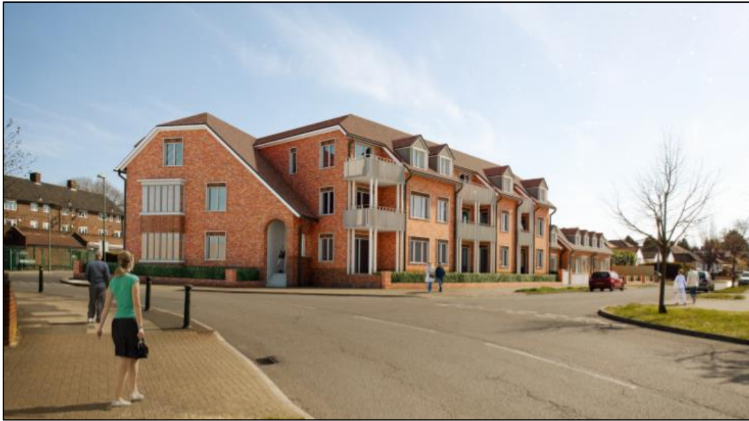
Fig.3. Computer generated image (CGI) - view of the proposal from the junction of Charterhouse Road with Winchester Road.
